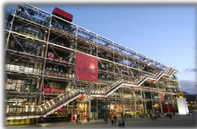
Gambar 2 : Exposed Structure
